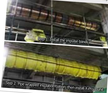
Step 1: Install the impulse bands
