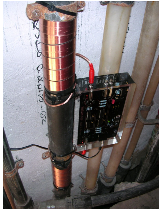
Vulcan S10 - Cold water main pipe
