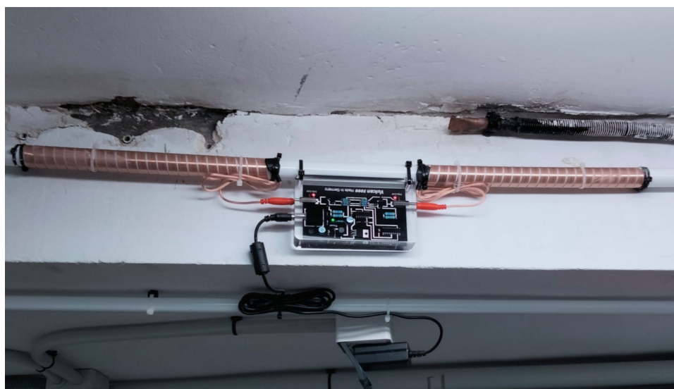
Vulcan 5000 at coldwater main pipe
